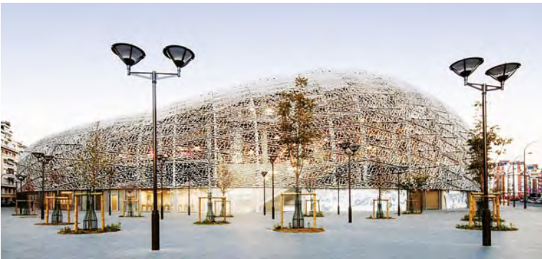
↑ In 2014, Briand wrote West is the Best , an exploration of the links between surfing and design, based on his travels in California. → A system of moulds was used to fabricate the concrete shell of Rudy Ricciotti's Stade Jean Bouin in Paris.
